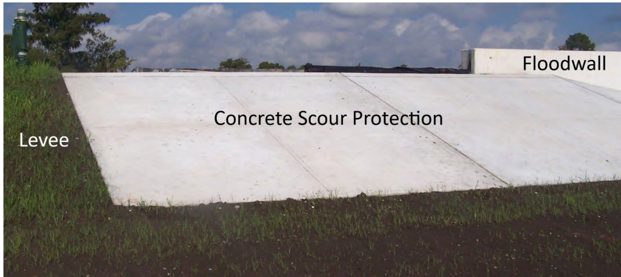
Figure 9: Illustration of Scour Protection at Levee-Floodwall Tie-in.
