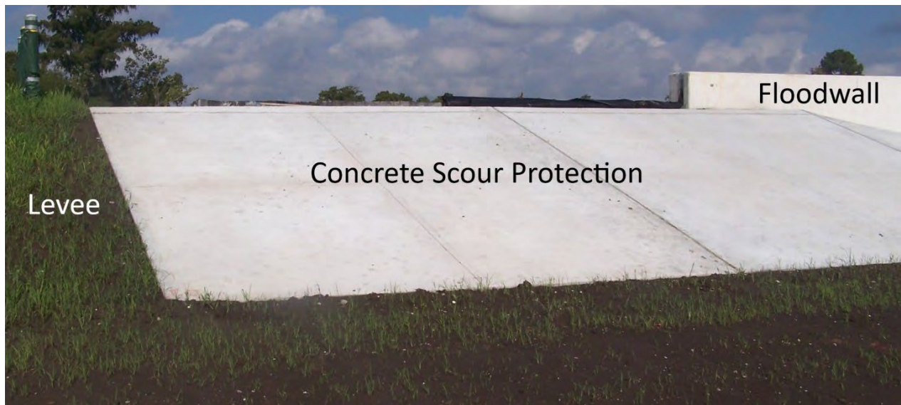
Figure 11: Illustration of Scour Protection at Levee-Floodwall Tie-in.
