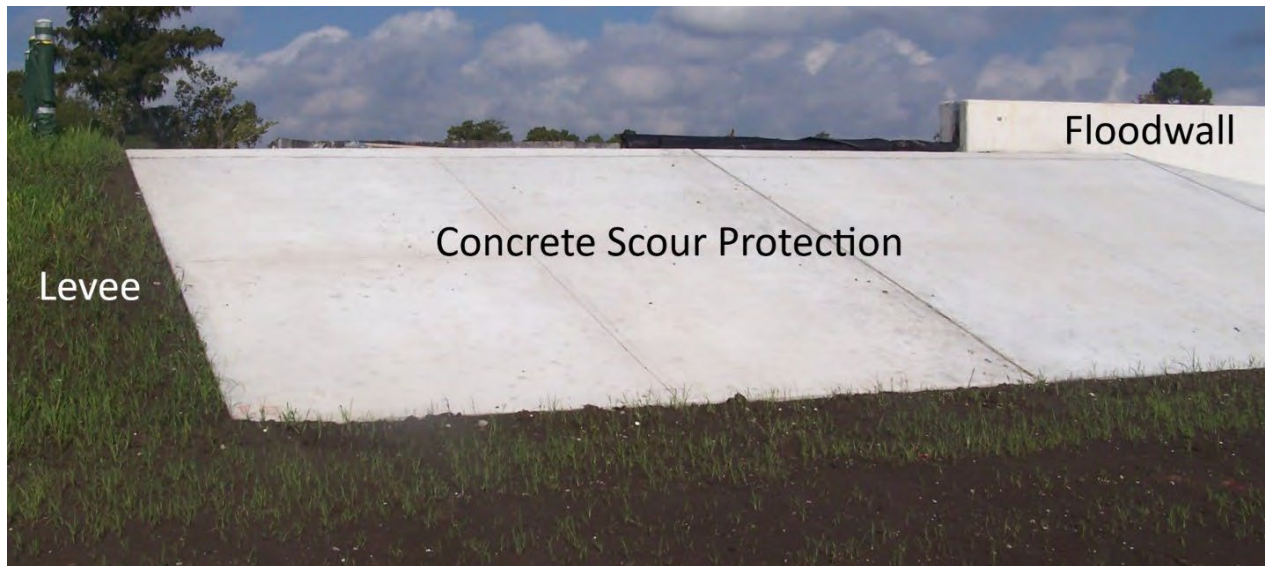
Figure 11: Illustration of Scour Protection at Levee-Floodwall Tie-in.
