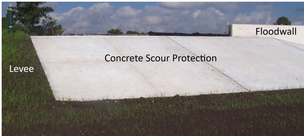
Figure 9: Illustration of Scour Protection at Levee-Floodwall Tie-in.
