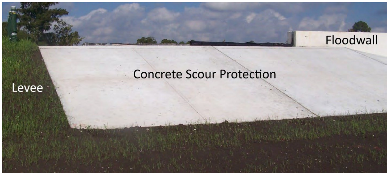
Figure 9: Concrete Scour Protection Example
