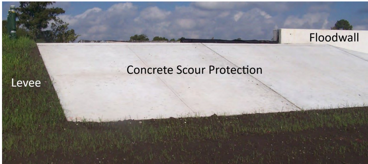
Figure 11: Illustration of Scour Protection at Levee-Floodwall Tie-in.
